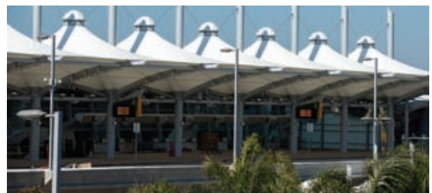
The dual-level roadway.
