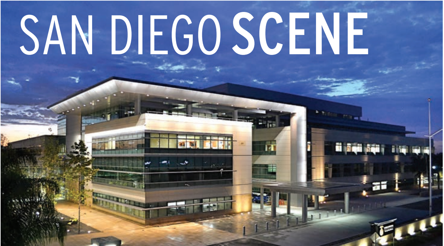
Naval Hospital at Camp Pendleton.
